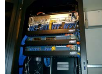
New EEC Network Installation
