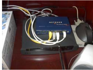
Old EEC Network Installation
