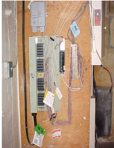
Existing Telephone Wiring Termination Installation
