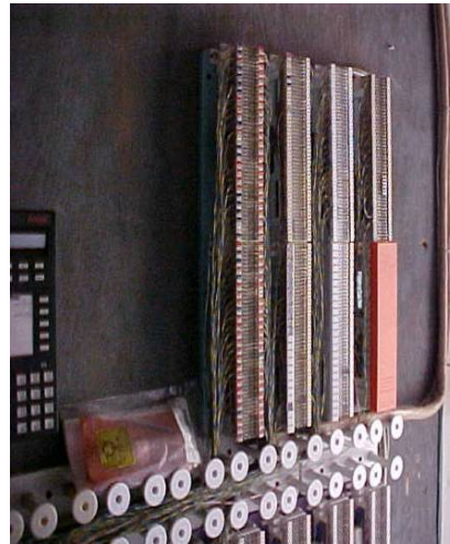
New Telephone Wiring Termination Installation
